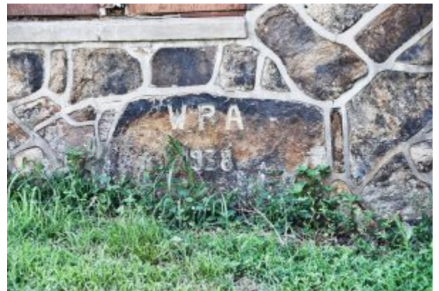
Stonework at the high school gymnasium at Menifee (Conway County).
