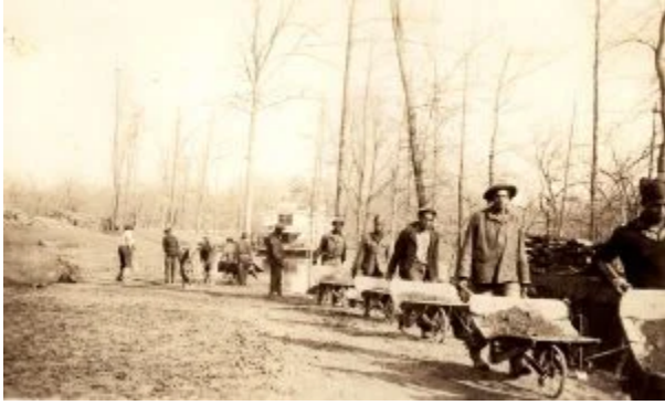
CCC enrollees using wheelbarrows at Jacks Bay; circa 1936.
